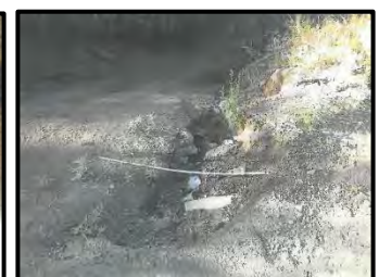
Erosion at the NW
