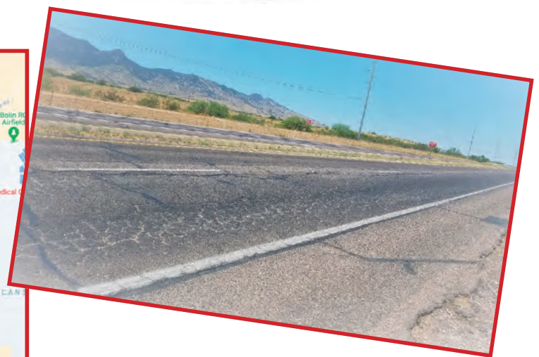
Buffalo Solider Trail disintegrating roadway surface
