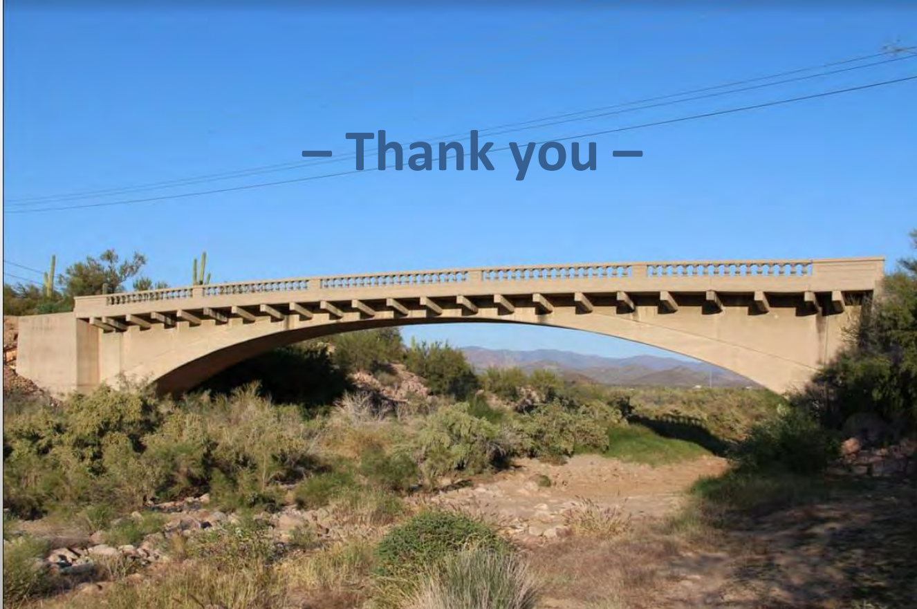
Queen Creek Bridge Pinal County
